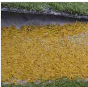
Defective seam
